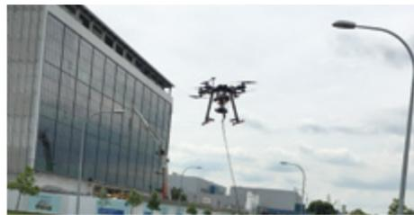
◀ Drones allow enforcement officers to inspect tall structures, inaccessible or unsafe workplaces
