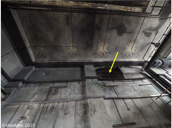
**Photograph 19:** Soot wash marks showing that the sprinklers had activated. Note the hole in the party wall between units 32E and 32F.
