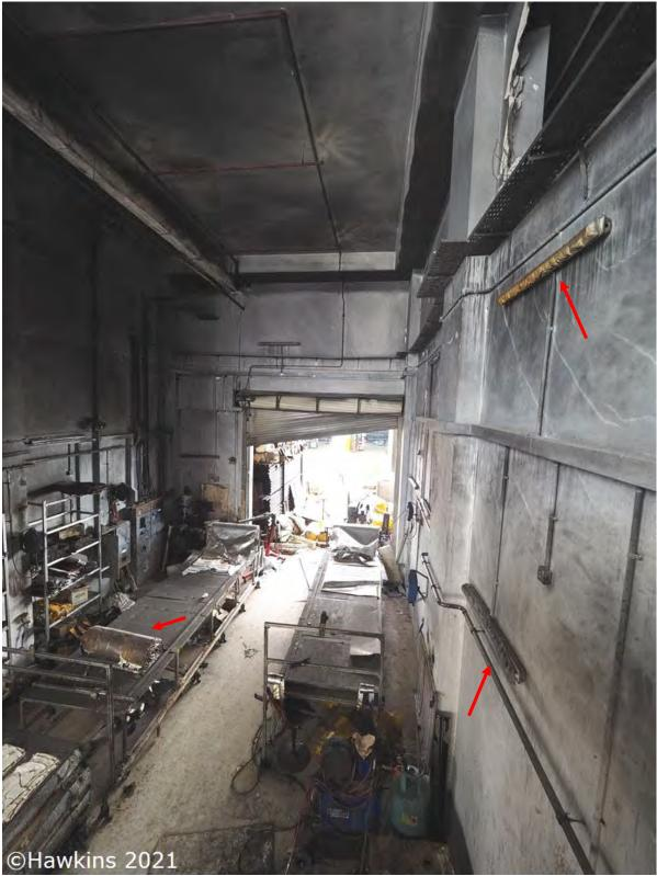
**Photograph 18:** Looking from the mezzanine to the roller shutter. Note there is no evidence of sustained fire damage, only scorching, blistering and superficial melting of papers, plastics etc.
