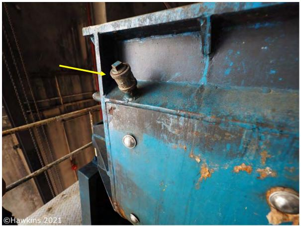
**Photograph 32:** One of the oil reservoir filling points. Note that it is capped.
