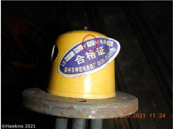
**Photograph 42:** The heating elements were each rated at 5kW.
