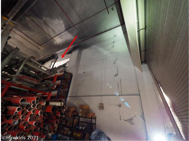
**Photograph 14:** Overview of the damage to Unit 32F. Note the hole and cracks in the party wall, the displaced roller shutter and the sprinkler wash on the ceiling.
