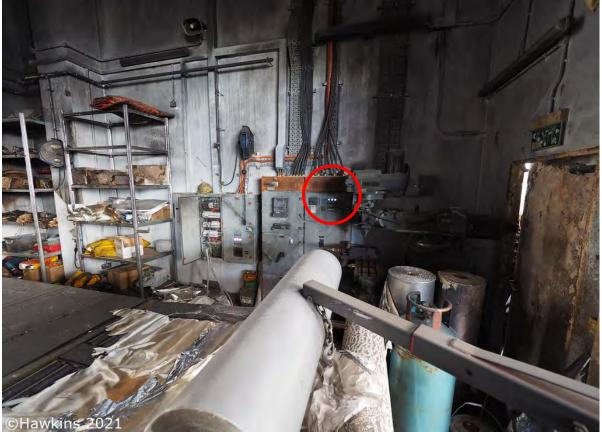
**Photograph 16:** Just inside the roller shutter, looking towards the electricity intake equipment. The items are heat damaged. Note the unburnt items on the shelving and the indicator lights of the electrical intake are illuminated.
