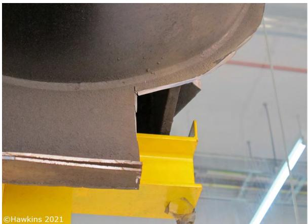
**Photograph 48:** The inside of the oil reservoir looking upwards to the underside of the reaction vessel at the location of the corner closest to the control panel. The soot deposits and the 'double skin' repair can be seen.
