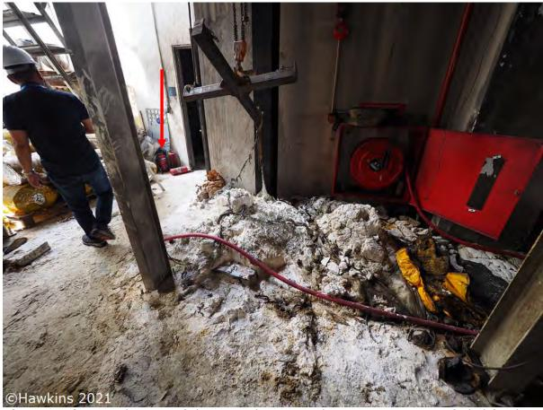
**Photograph 22:** The rear of the unit adjacent to the mezzanine. An unfurled fire hose can be seen along with some fire-extinguishers, two of which had been discharged.
