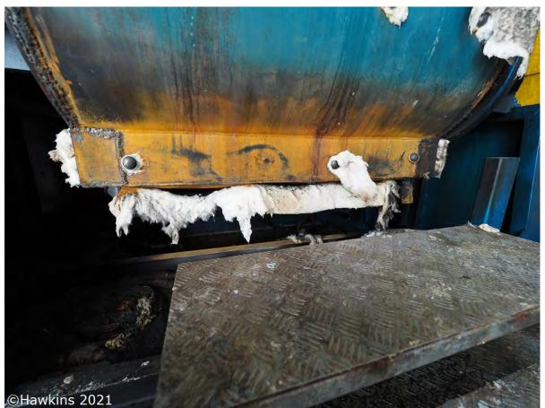
**Photograph 35:** The casing of the machine was rusty at low level on one side of the oil reservoir.
