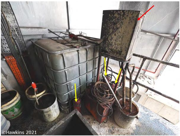
**Photograph 24:** The IBC, water pump (red arrow)and fire extinguishers (yellow arrows) on the mezzanine.
