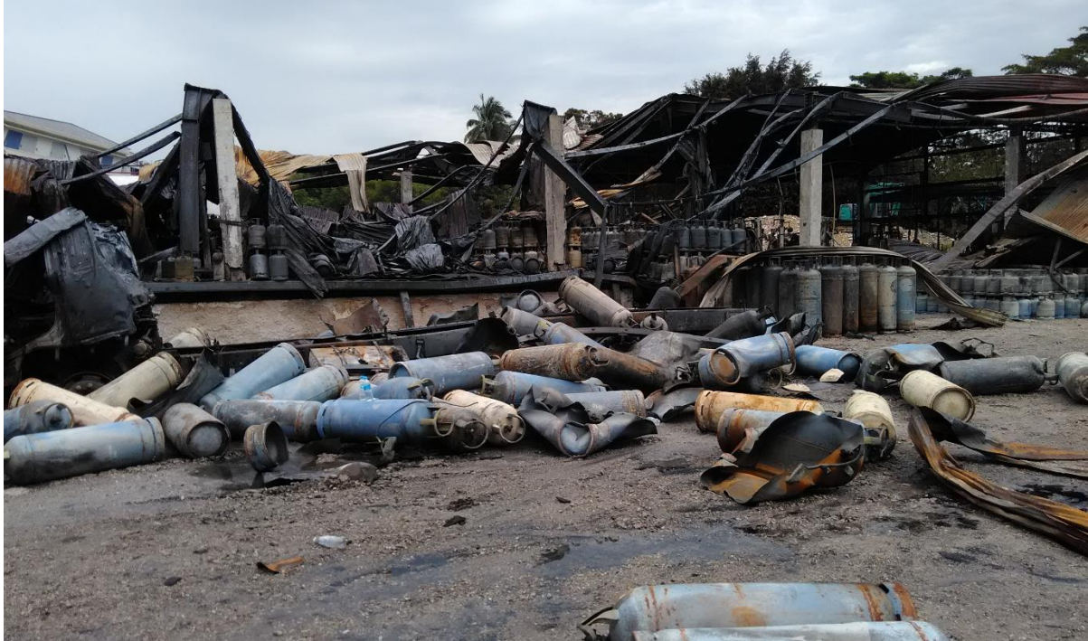
Figure 2. Scene of the filling shed after the fire
