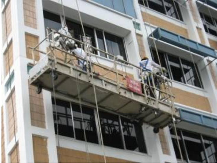
Photo showing a typical gondola used in painting of a building
