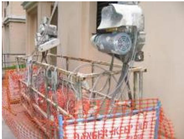
Photo showing the winches used for the climbing of the gondolas
