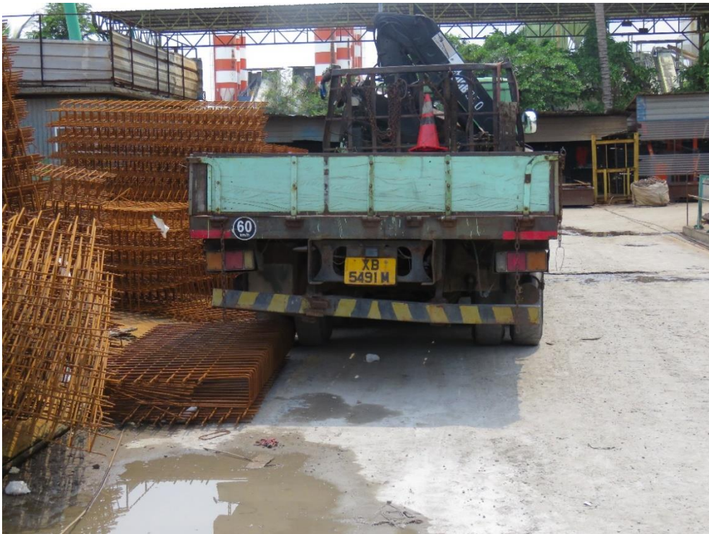
Images 2 and 3: Lorry Loader Attached with Hydraulic Crane Arm
