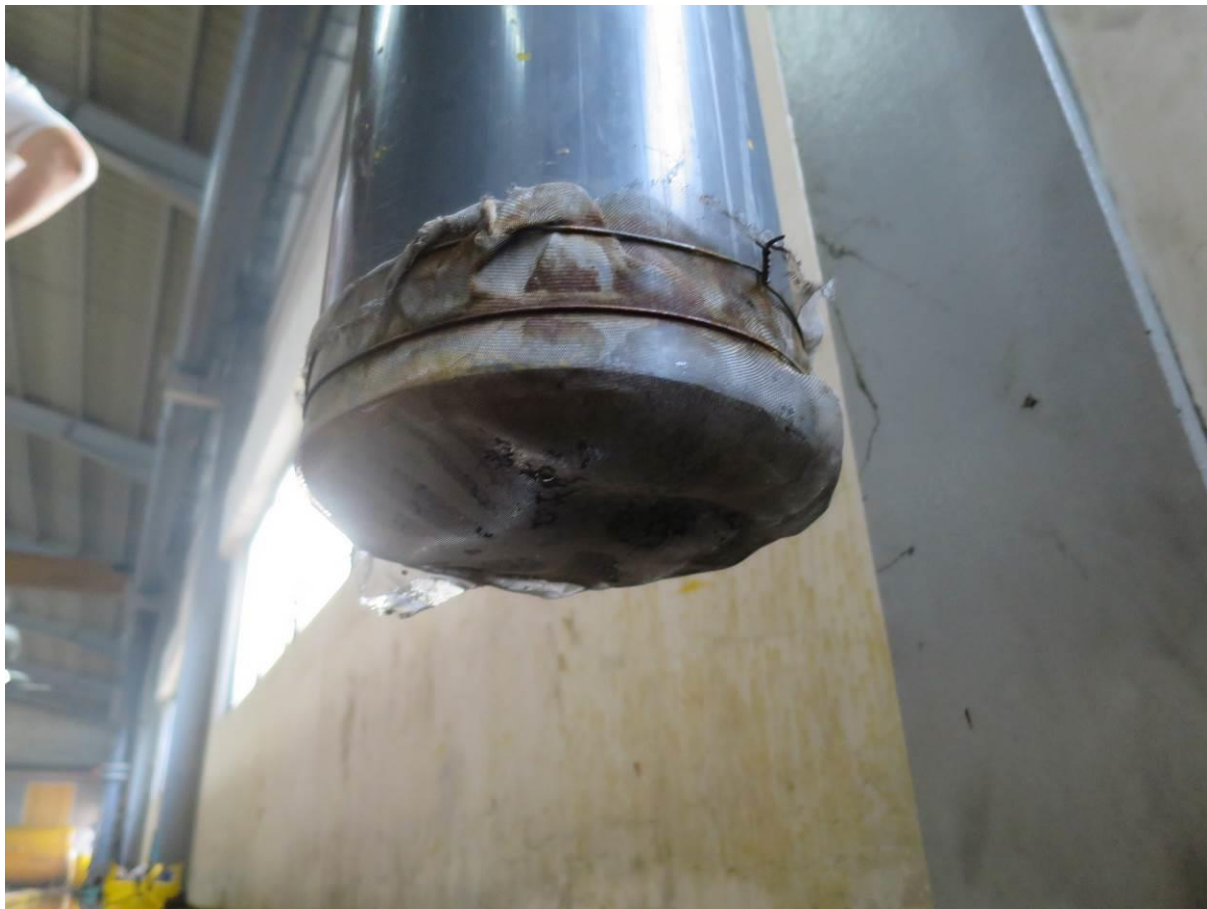
Photograph showing the mesh filter screens used on suction pipe intakes
