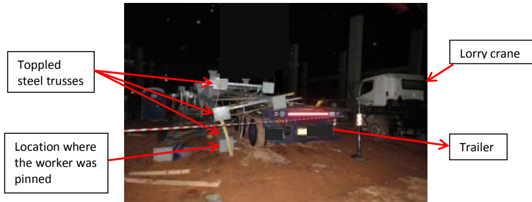
Overview of the accident site (Photograph taken in the night of the accident)
