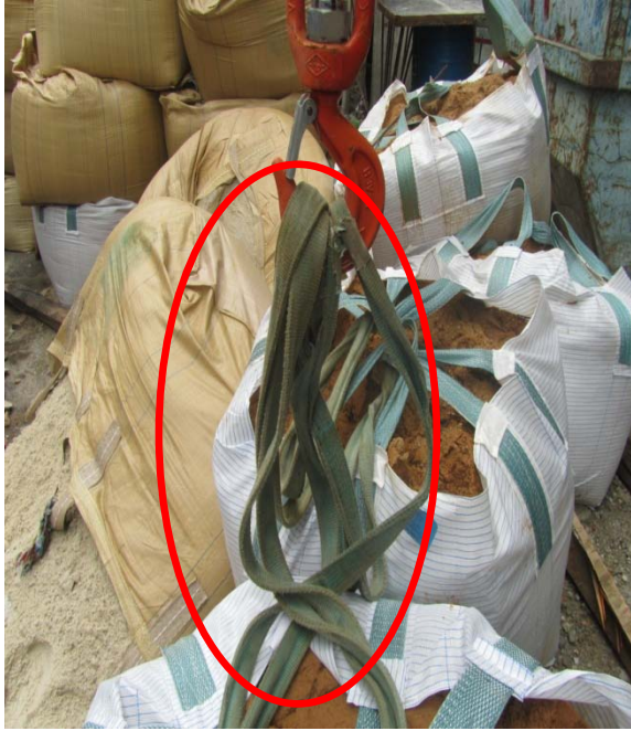
Figure 8 Lifting Gears found to have no identification tags and certifications. Such tags and certifications are necessary to ensure that only lifting gears tested and examined by Authorised Examine
