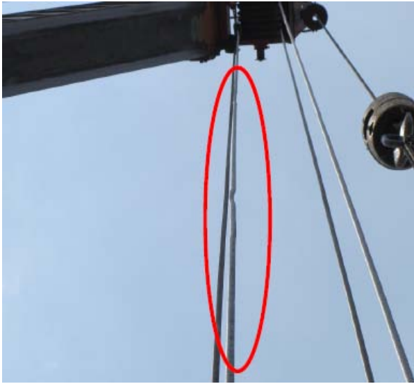
Figure 2a A kinked wire rope of a crawler crane. This is a permanent damage to the wire rope which results in a loss of strength to the rope.
