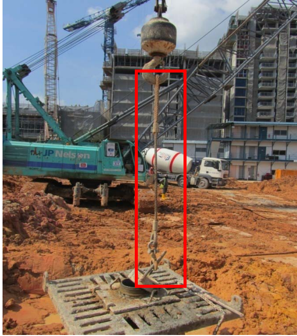
Figure 8 Lifting Gears found to have no identification tags and certifications. Such tags and certifications are necessary to ensure that only lifting gears tested and examined by Authorised Examine
