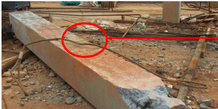
Figure 7 - Defective and kinked Lifting Gear
