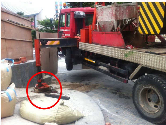
Figure 6 - No Lifting Plan and PTWS for lifting operation involving a Lorry Crane
