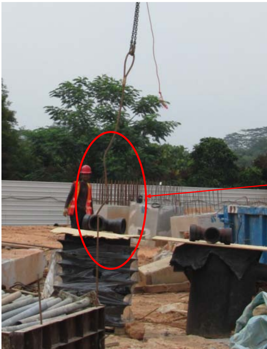
Figure 11 - Defective Lifting Gear - Multiple Kinks
