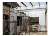
Unsafe means of access and egress between the  $2^{\rm nd}$  and attic levels of the building under construction.
