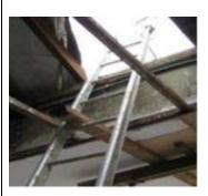
Unsecured ladders were used for access to work areas on the roof top.
