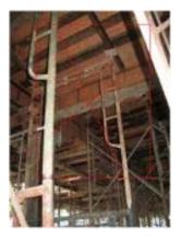
Unsafe structures used to support parts of the building under construction (formwork shoring) which exposes workers to the risks of collapsing structures
