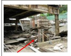
Poor housekeeping at the work site which exposes workers to the risks of being struck by falling/collapsing objects
