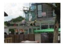
Workers were seen working at height without proper fall protection and anchorage points for safety harness.
