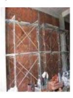
Access ladder, guard rails and toe-board were not provided to allow safe access to work platforms and prevent falls from openings.
