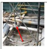
Scaffold was not erected on solid foundation exposing it to the danger of collapsing
