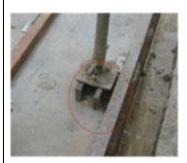
Scaffold not erected on sound foundation exposing it to the danger of collapsing.
