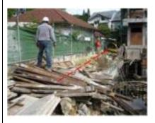
Lack of a proper walkway exposing workers from falling hazards and impaling hazards from exposed sharp objects.
