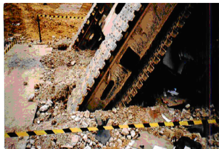
Figure 10: Collapse of crane due to inadequate steel plates coupled with soft ground condition
