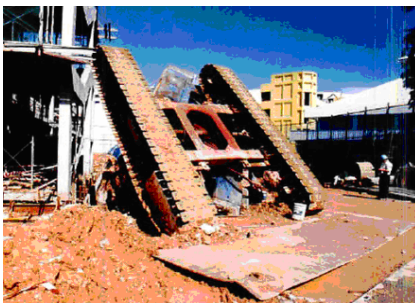
Figure 10: Collapse of crane due to inadequate steel plates coupled with soft ground condition
