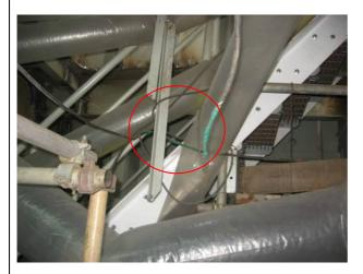
Failed to ensure that all electrical connections are in accordance with accepted principles of sound and safe practice. Electrical wires were branched out with improper methods.
