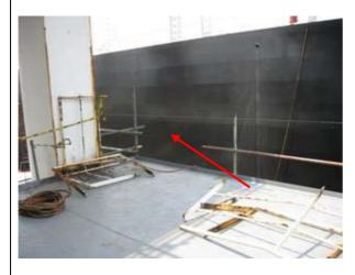
Failed to provide effective barriers to prevent falls through open sides from which a person might fall more than 2 metres
