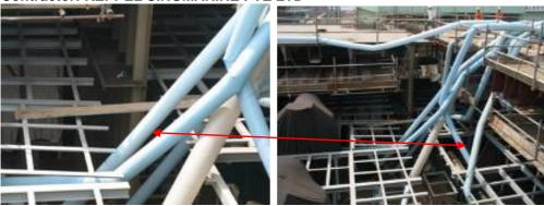
Failed to provide safe means of access and egress for scaffold erectors erecting the hanging scaffold
