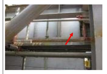
Failed to provide effective barrier on every side of the work platform from which a person might fall more than 2 metres
