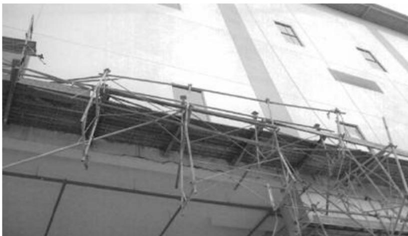
**Figure 8:** Poor working platform
