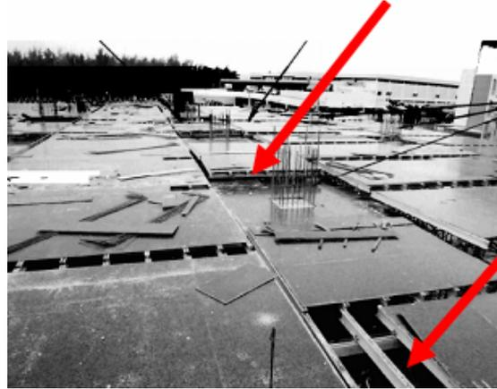
Figure 10: Lack of covering for open penetration (indicated by the arrows)
