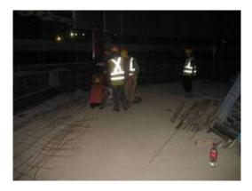
Photos taken with flashlight by the OSH Inspectorate revealed that workers were working with insufficient lighting in that area.
