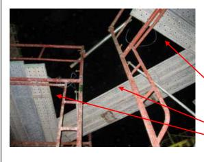
Failure to provide every side of the work platform from which a person was liable to fall more than 2 metres with toe-boards and guard-rails
