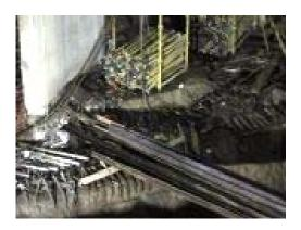
Failure to keep the passageways and places of work, free from debris and protruding objects that could cause tripping.
