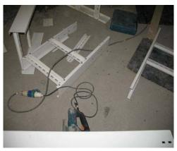
Failure to ensure that the electrical extension cable used to connect the electrical cutter shall not be left on the ground unless it was provided with adequate protection to withstand the wear and tear to which it may be subjected to.
