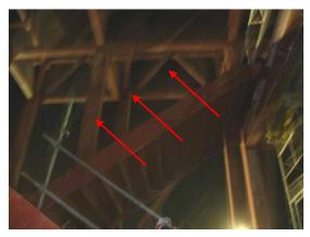
Failure to provide and maintain handrails on one side of the staircases at multiple locations
