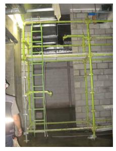
Failure to provide every side of work platforms with guardrails and toe-boards.
