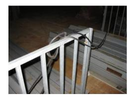
Failure to ensure that all electric wiring was supported on proper insulators.
