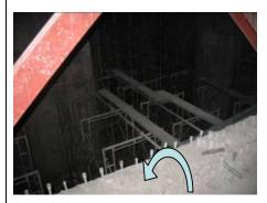
Failure to provide effective guard-rails , barriers or other equally means to prevent fall to open side or opening through which a person is liable to fall more than 2 metres
