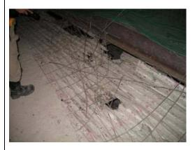
Gaps and corroded openings were found on the existing bondeck. Workers were seen stepping on the existing bondeck while working at the area.
