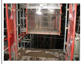
Failure to ensure that the interlocking device of the passenger hoist bearing was in good working condition such that the cage or platform cannot be moved away from the landing until the gate is closed
