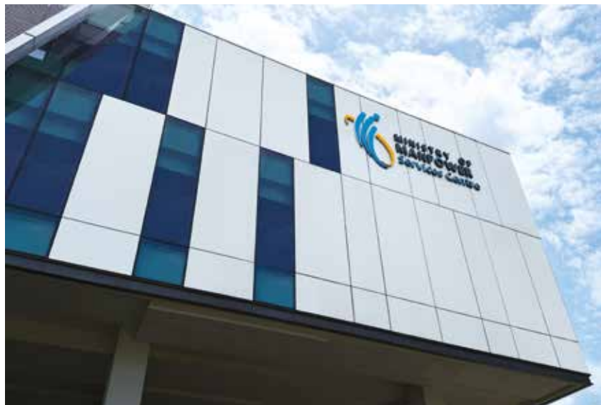
Opened in 2012, the MOM Services Centre on Bendemeer Road serves as a one-stop hub for employment-related services, offering an integrated service experience for both employers and workers. (Photo credit: MOM)
