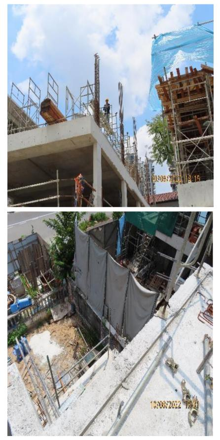
A worker was seen performing work at the edge of the third floor of the structure, without barricades or a fall arrest system. The worker was not wearing a safety harness.
