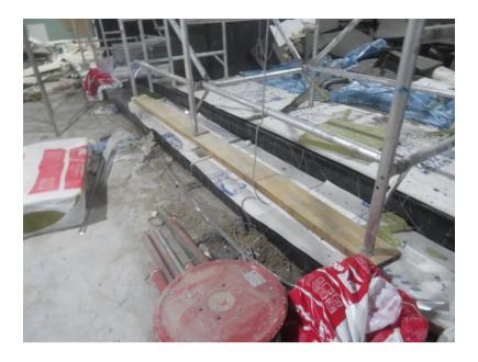
Some of the scaffold structures were erected on void areas, whereas others were placed on unstable foundations.
