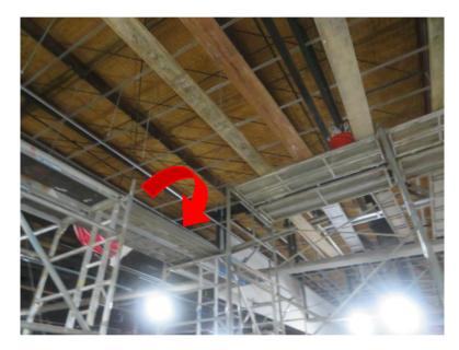
Toe-boards and guardrails were not provided on the sides of the work platform where workers could fall from more than 2 metres of height.
