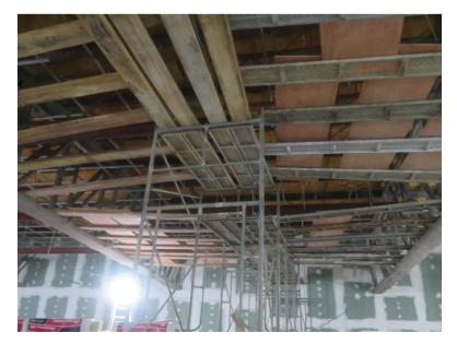
Workers were found working on work platforms that were not closely boarded and properly secured, which may lead to accidental displacement (i.e. shifting of the platform).
