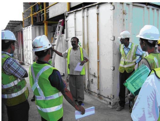
Briefing workers before compressed air work
