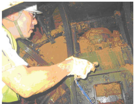
Working in cutter head chamber
