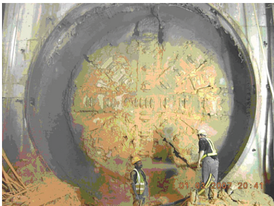
TBM cutter head
