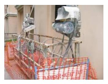
Photo showing the winches used for the climbing of the gondolas
