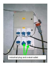
Fig. 1 – This photograph shows a wall mounted SOA with uncluttered electrical cables connected to industrial socket-outlets using industrial plugs. All live parts are fully enclosed.
